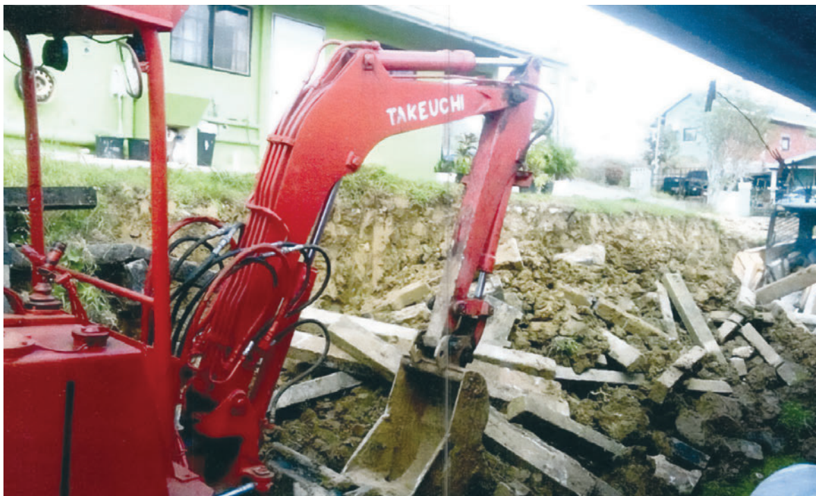
REMOVAL OF CRIB WALL (AFTER)
