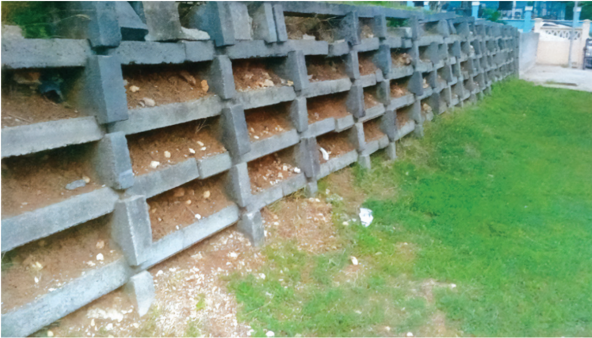
MS. T'S CRIB WALL TO BE REMOVED (BEFORE)
